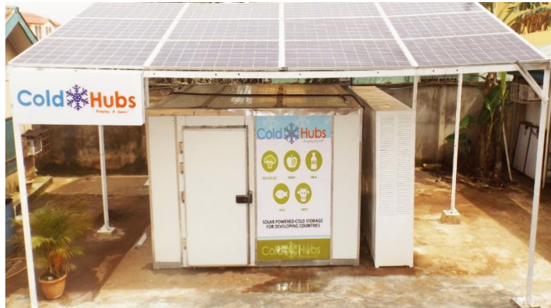
Figure 7: ColdHubs: A solar-powered, walk-in, modular unit for storing fresh produce in Nigeria. Source: Ikegwonu (2020).
